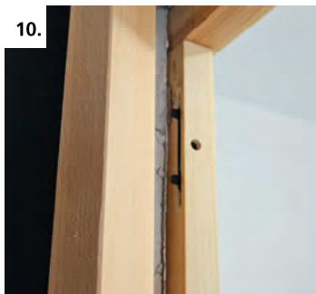
Hinge the jamb leg into place behind casing, using beveled edge against pocket door
