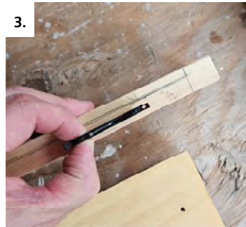
Determine slot position in jamb and casing
